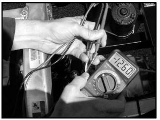
Figure 11b-41 Bed Lift Motor Voltage Reading with Switch in DOWN position
