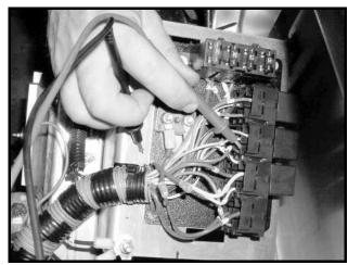
Figure 11b-13 Differential Relay Coil Circuit Test
