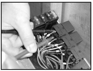
Figure 11a-12 Start Relay Coil Circuit Test
